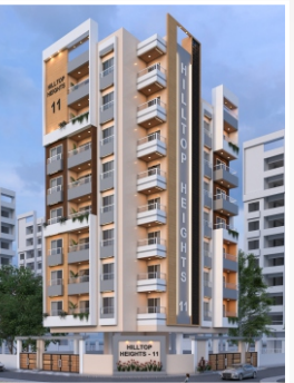
HILLTOP HEIGHTS - 11 (Hilltop, Ram Nagar) Ongoing
