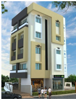
SIDDHIVINAYAK RESIDENTIAL - I (Zingabai Takli) Completed
