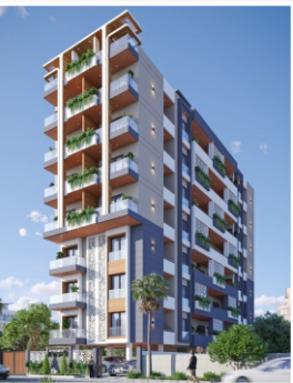
HILLTOP HEIGHTS - 14 (Hilltop, Ram Nagar) Ongoing
